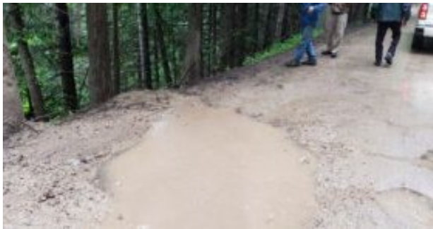
Sediment laden runoff from FSR 437 draining directly into Hayden Creek
