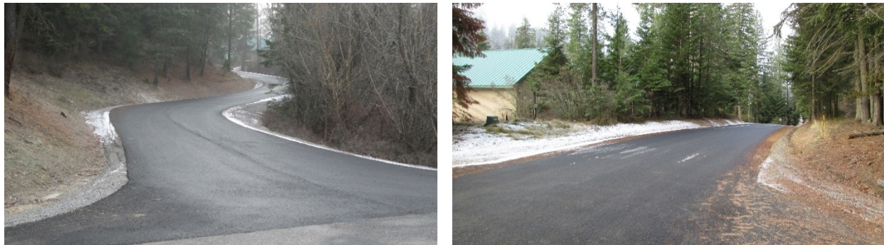
Two views of one- tenth mile of Mokins Bay Road paved to reduced sediment yield.
